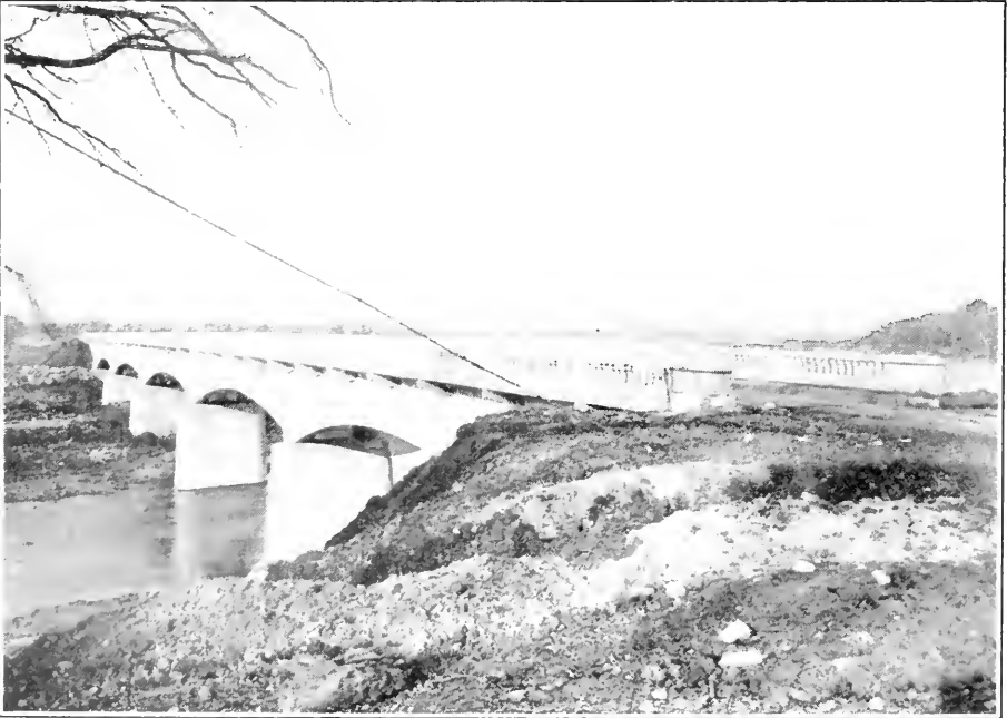
View of the New Cockshutt Bridge, Showing Rip Rap on the Approach.
